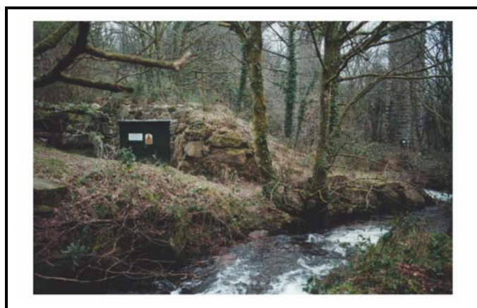
Hydroelectric powerhouse near Helston, buried to reduce impact 145kW
