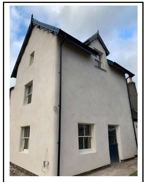
Hempcrete external solid wall insulation on Listed Building
