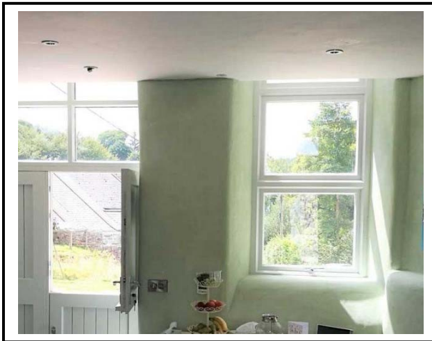
Hempcrete internal solid wall insulation Cardinham
